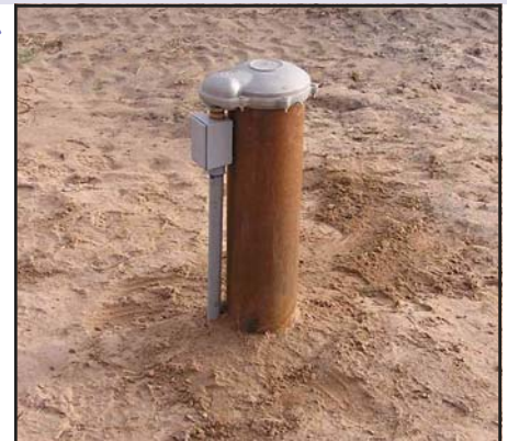
Standard domestic water well in Weld County
